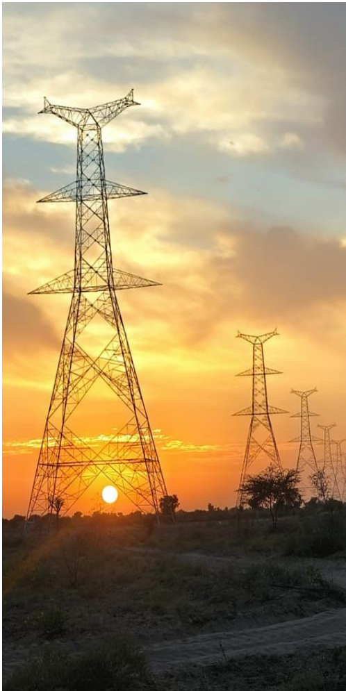
765KV D/C Merta II - Barmer Transmission Line
