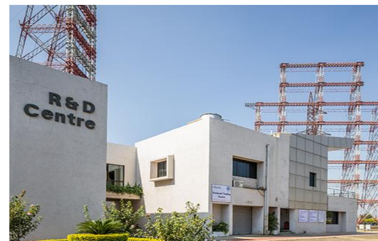
Tower Testing Facility
