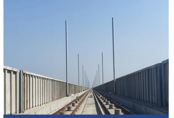
Over Head Electrification Masts for Mumbai-Ahmedabad Bullet train corridor
