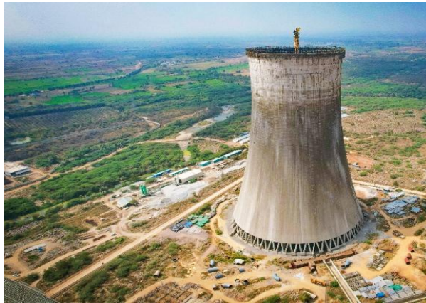
India's 2 nd Largest Cooling Tower (Yadadri) – 199 mtr
