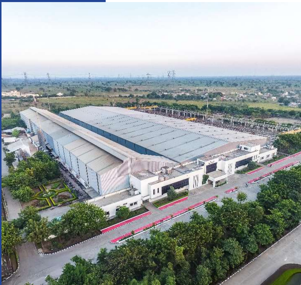
Deoli Tower Factory
