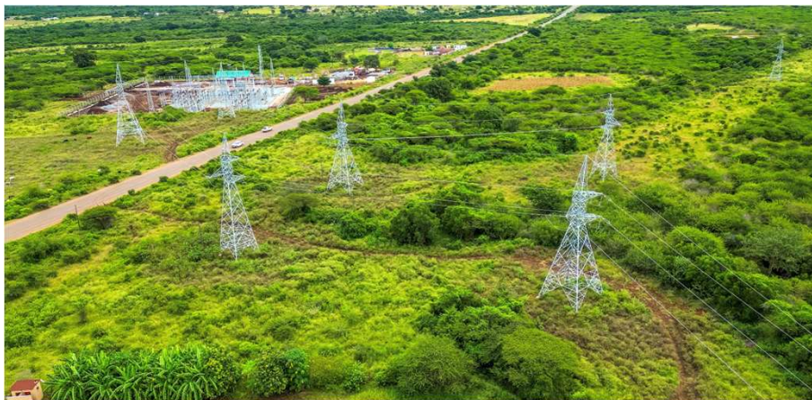
Eswatini 132kV Transmission Line Project
