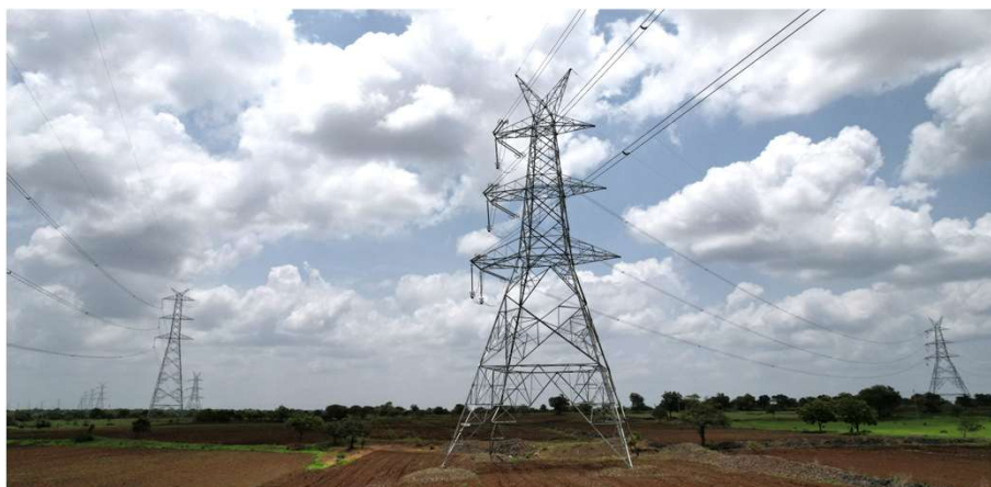
400kV Transmission line project in Solapur, Maharashtra
