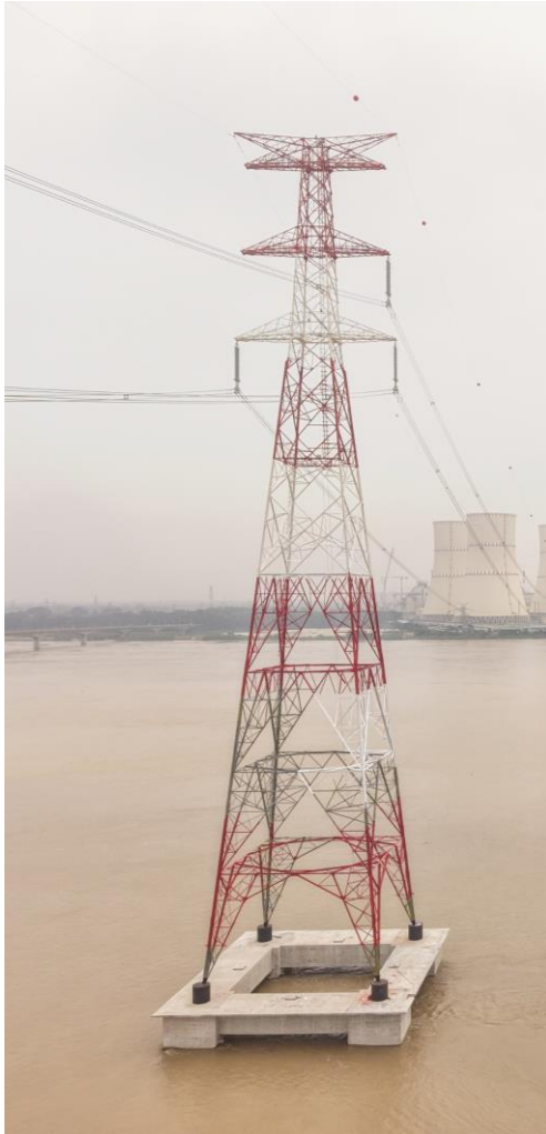
400kV D/C Rooppur-Gopalganj Transmission Line
