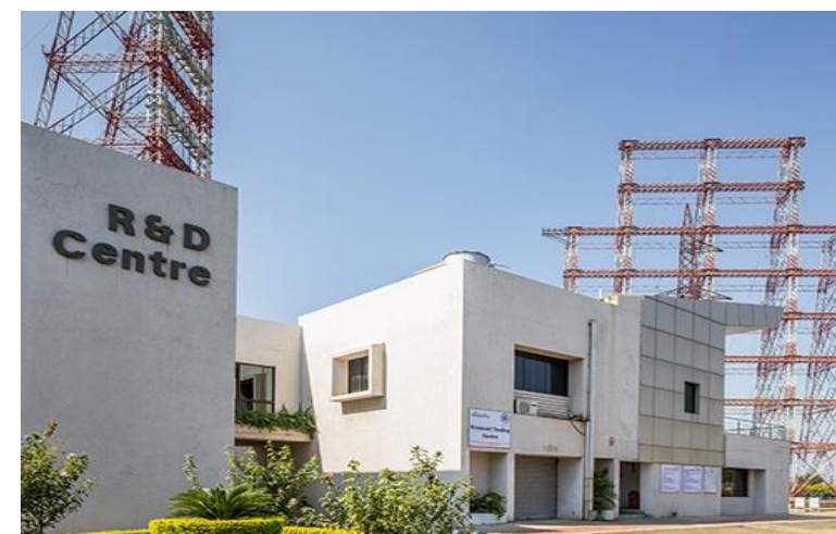
Tower Testing Facility
