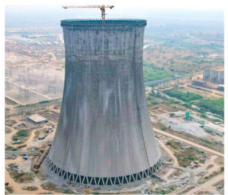
Cooling tower at Udangudi and Yadadiri
