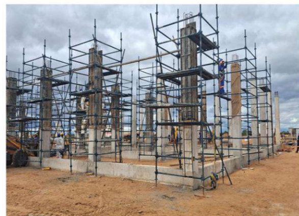
400kV Mmamabula Substation project (Botswana)
