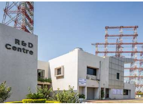
Tower Testing Facility - Deoli
