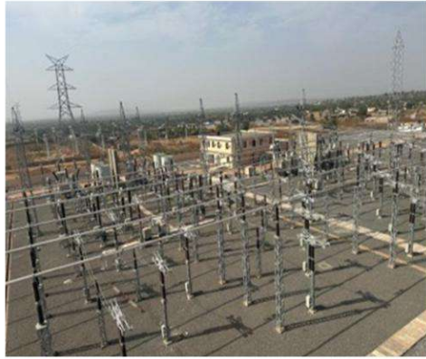
225/30 kV Substation project at Mali
