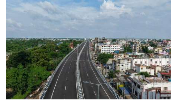
Begusarai elevated road project, Bihar
