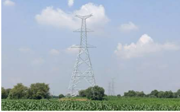
Koppal-II PS – Narendra 765 kV D/C line, Karnataka
