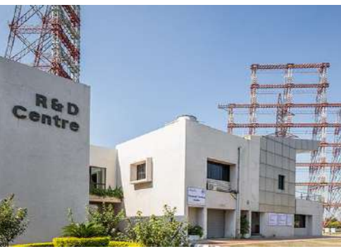
Tower Testing Facility - Deoli
