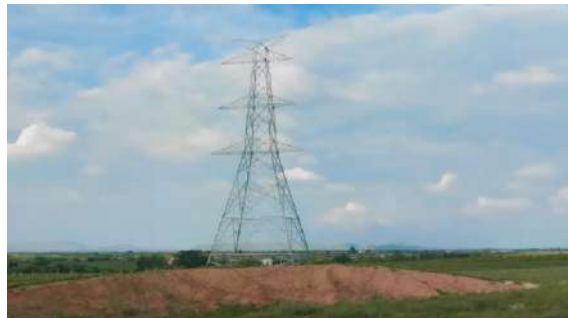
765KV D/C Dausa-Ghiror TL project, Rajasthan
