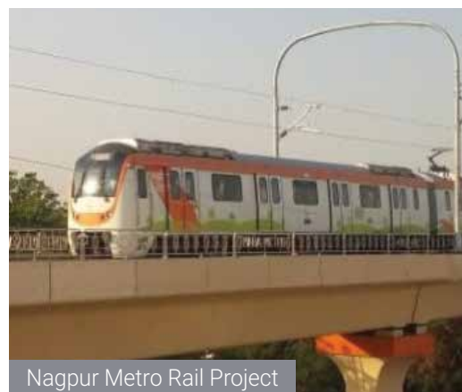
Nagpur Metro Rail Project
