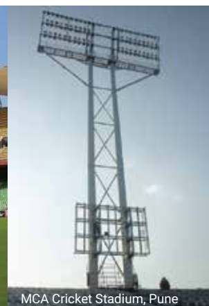
MCA Cricket Stadium, Pune
